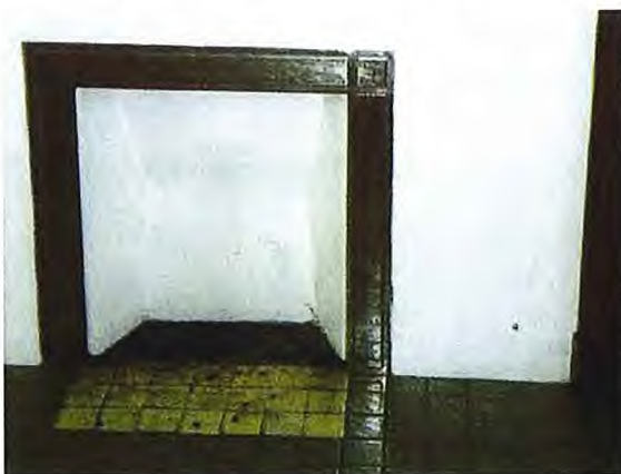
Figure 1: Asbestos-containing material was commonly used around fireplaces
